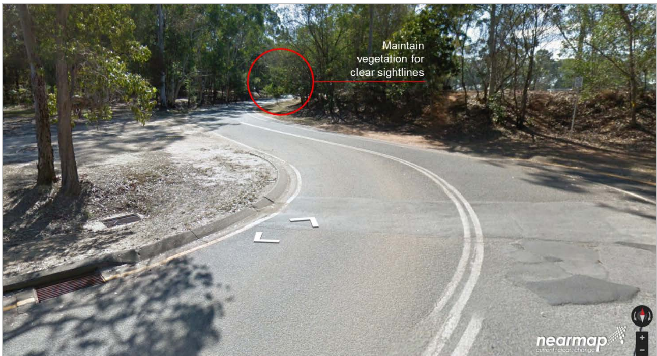
Figure 1-2 Existing Internal Road (view from right turning vehicle into temporary road looking north)
