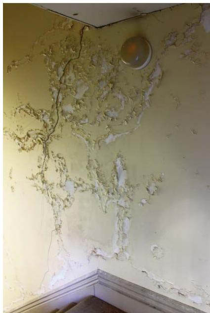
Figure 16 – Showing Internal Cracking and Peeling of Paint
