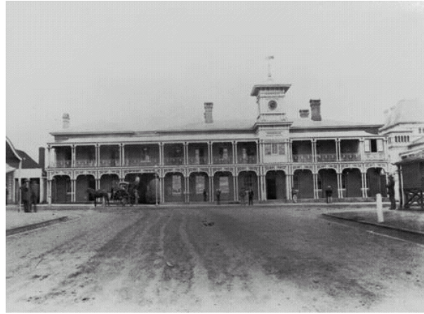
Figure 10 - Lands and Works Office (SLQ ID 44355)
