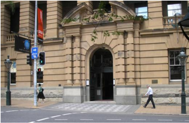
Figure 36 – Gas Lamps – George Street (Urbis 2017),
