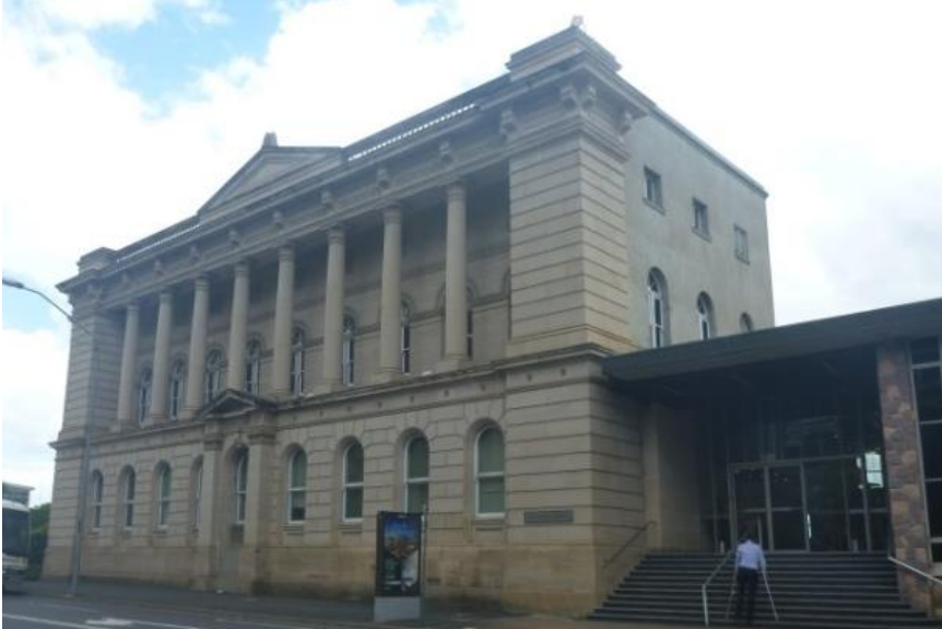
Figure 27 - The Former State Library (Urbis 2015)
