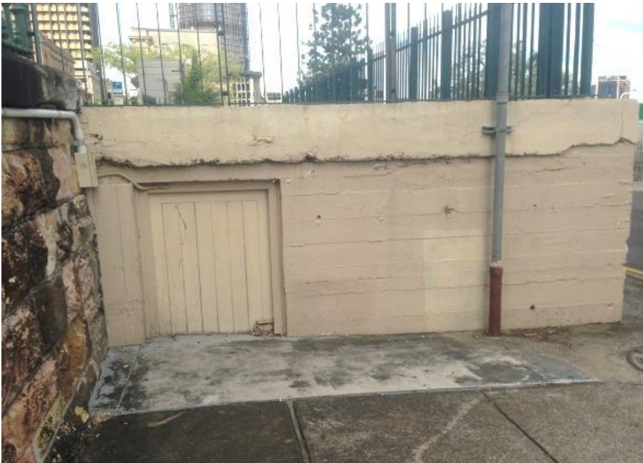
Figure 32 - Partial View of Air Raid Shelter, Western Elevation (Urbis 2016)
