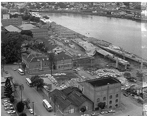
Figure 23 – Construction of the Riverside Expressway 1972
