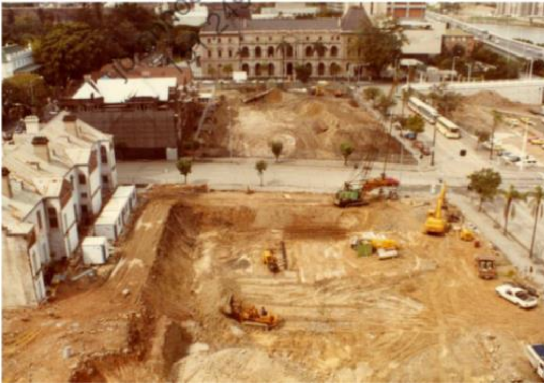
Figure 19 – Clearing Behind Harris Terrace and The Mansions In 1983
