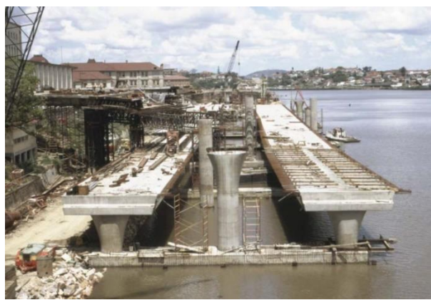
Figure 22 – The Riverside Expressway under construction
