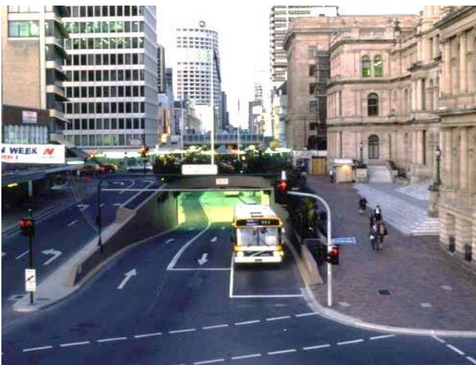
Figure 20 – Queen Street bus tunnel shortly after opening, 1989
