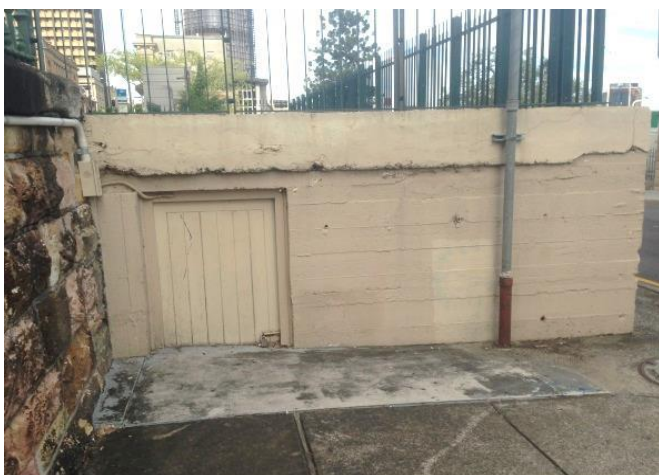
Picture 39 - Partial View of Air Raid Shelter, Western Elevation
