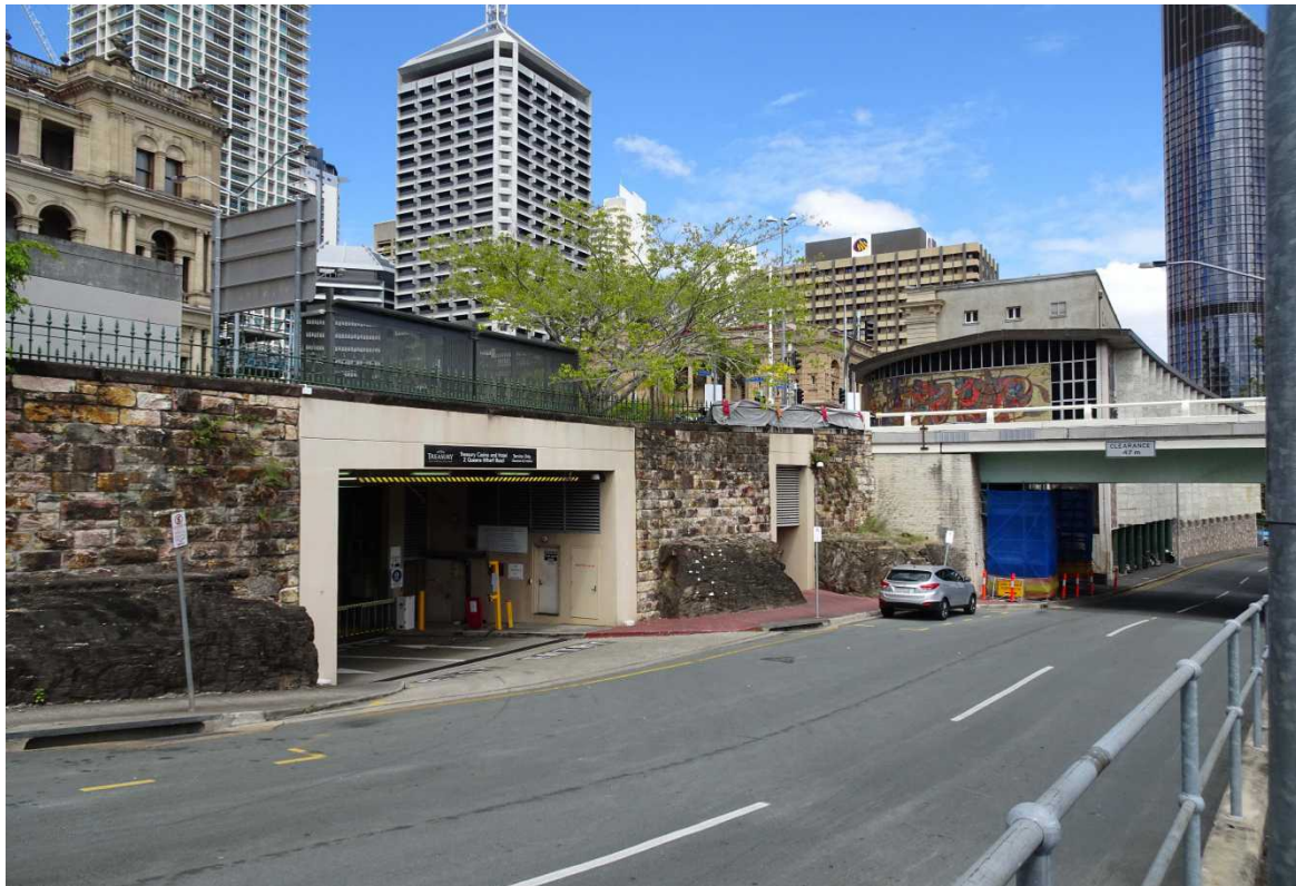
Figure 7: Modern driveway and former closet recess, from west (EHP, 2016)
