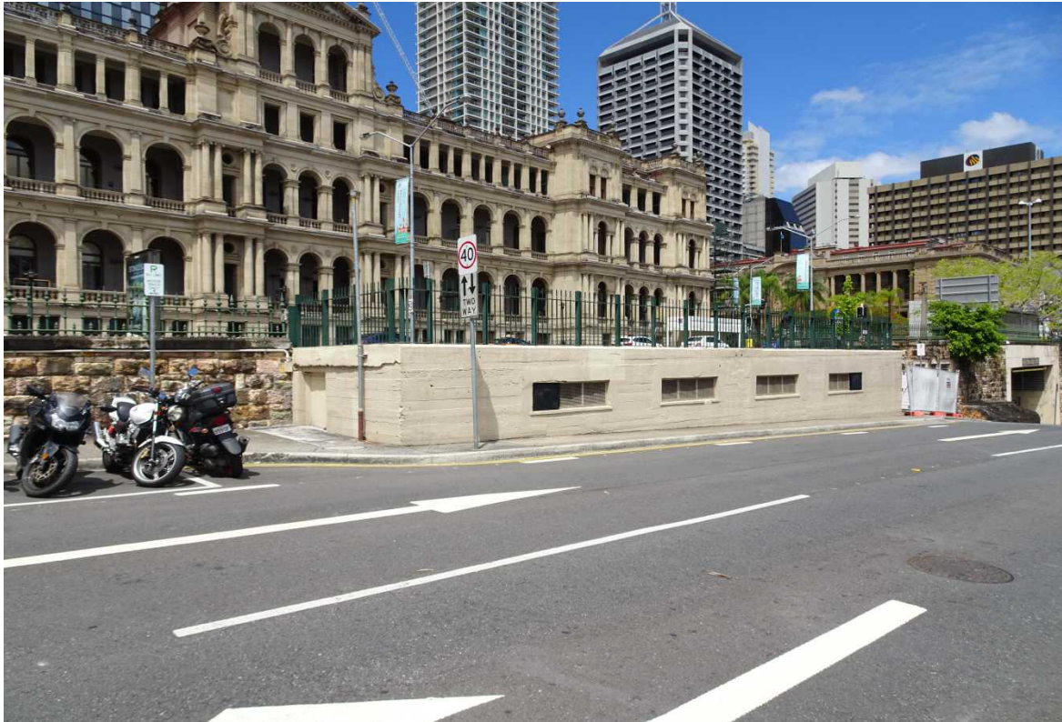
Figure 5: WWII air raid shelter, from west (EHP, 2016)
