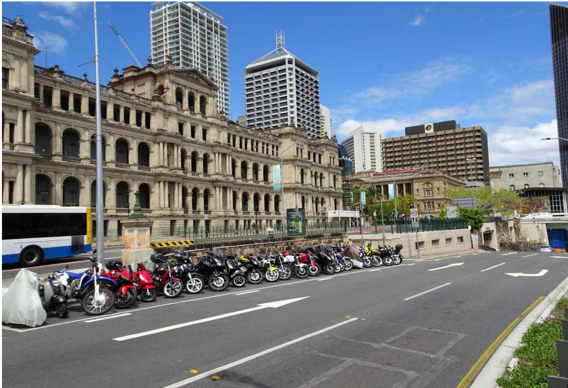
Figure 3: William Street retaining wall, from west (EHP, 2016)
