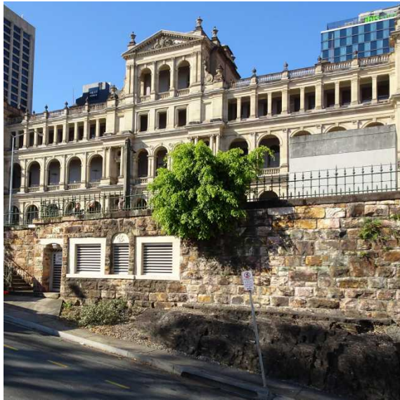
Figure 1: William Street and Queens Wharf Road retaining walls (EHP, 2016)
