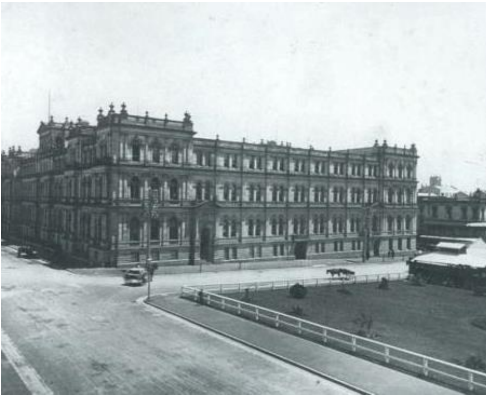
Picture 14 - The First and Second Stages of the Treasury Building (south view), circa 1904.
