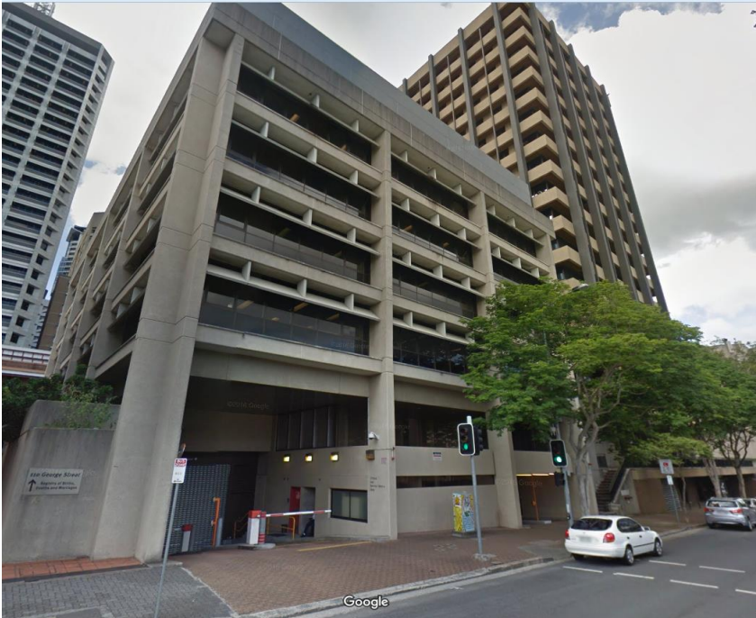
Picture 32 - Executive Building and Annexe
