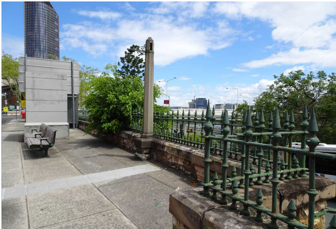
Figure 8: William Street parapet with interwar concrete ventilation shaft, from north (EHP, 2016)
