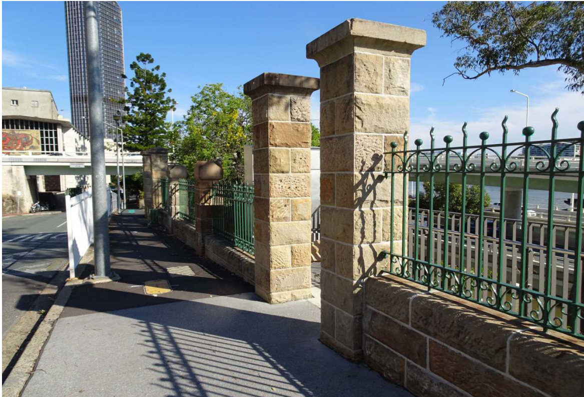
Figure 11: Gateway to former stairs, Queens Wharf Road wall, from north (EHP, 2016)
