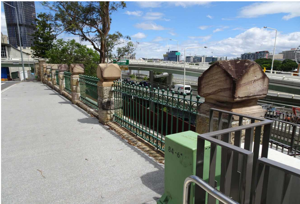
Figure 10: Queens Wharf Road wall, from north (EHP, 2016)
