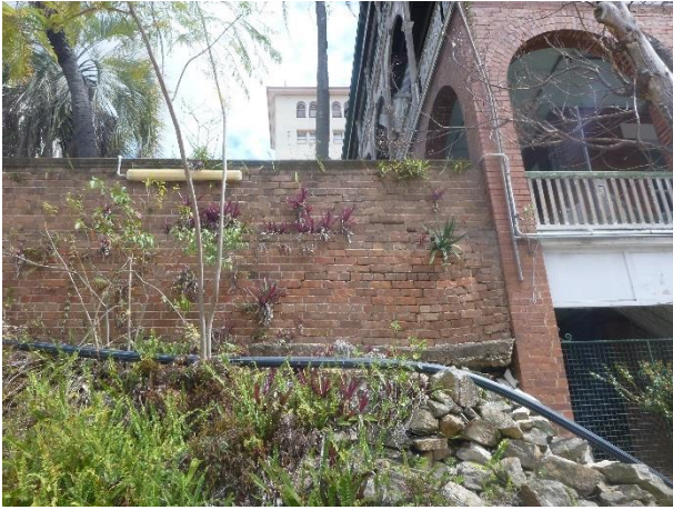
Picture 13 – Lady Lamington Nurses Home, masonry wall eastern side
