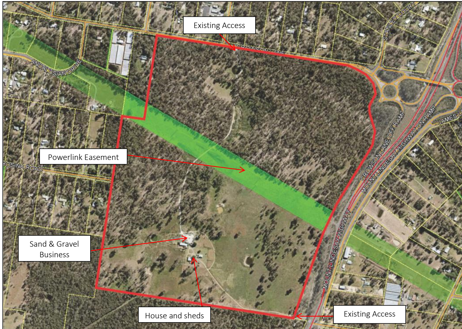
FIGURE 1: AERIAL PHOTOGRAPH OF THE SITE
