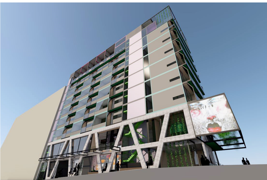
Wren Street elevation expressed structure
