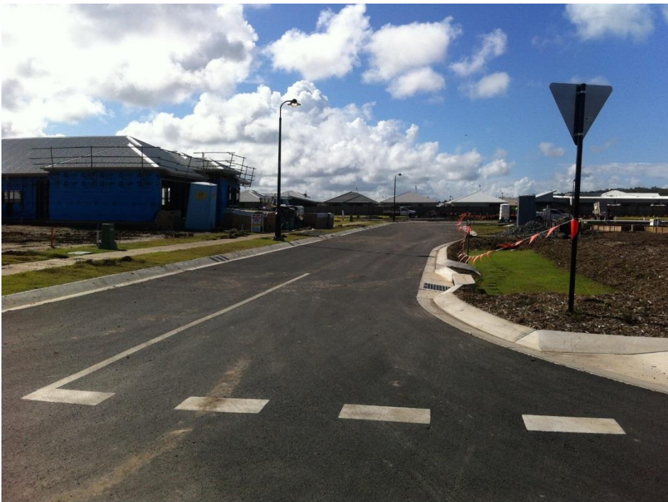
Photo: Example of biopod with one-way cross fall, pavement narrowed locally around biopod to create space for the biopod, treating a long stretch of road. Biopod with protective turf during house building.
