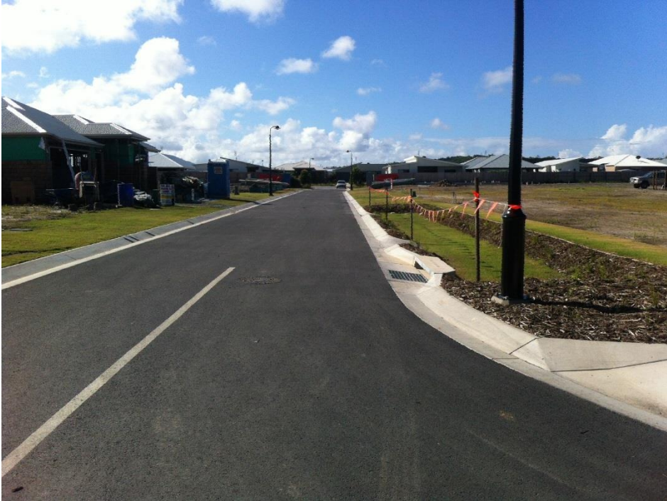
Photo: Example of biopod with one-way cross fall, pavement moved over to create space for the biopod, treating a long stretch of road. Biopod with protective turf during house building.
