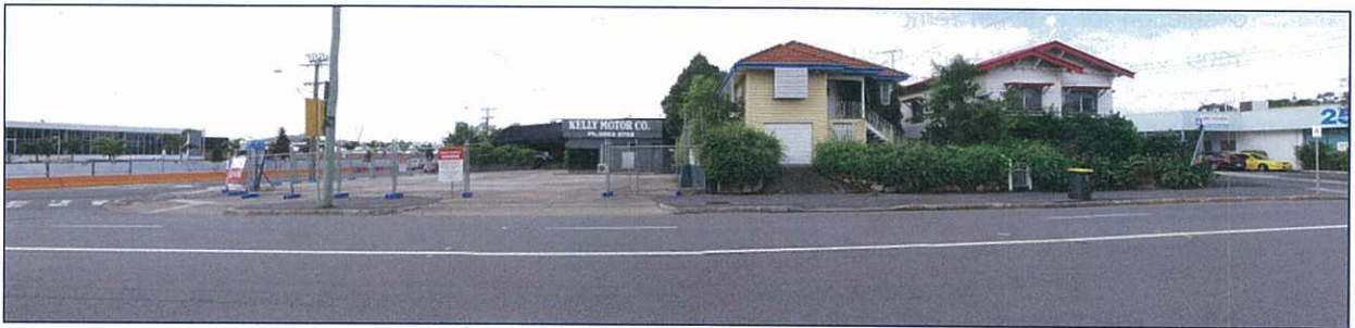
Photograph 4: Panoramic view of the site looking north-west to north-east from the southern side of Campbell Street
