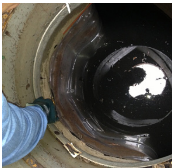
Inspection of the flexible separator skirt from inside the maintenance access wall opening.
