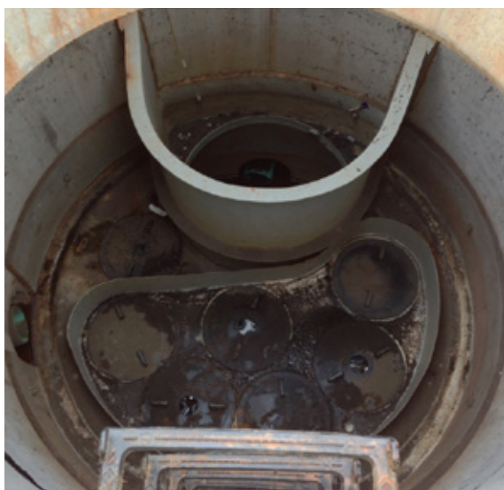
A view of the cartridge deck from the surface showing all the cartridge lids intact and no standing water on the deck.
