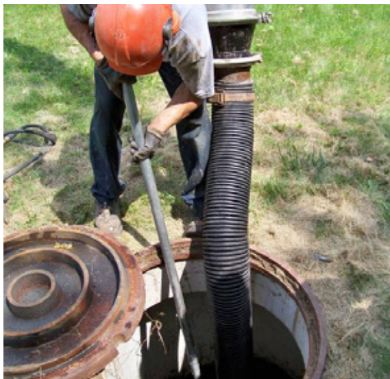
A maintenance worker stationed on the surface uses a vacuum hose to evacuate water, sediment, and floatables.
