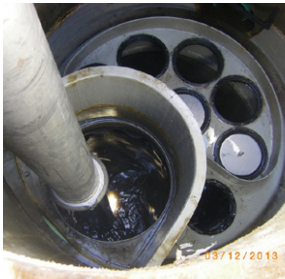
Vacuum wand inserted through the maintenance access wall opening.
