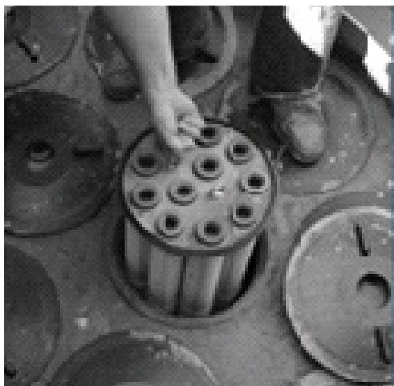
Installation of a filter cartridge into a cartridge receptacle in the deck.
