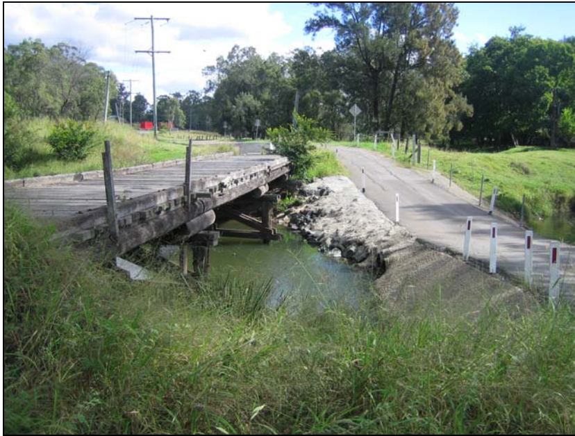
Photo 1 Patrick Street Bridge
