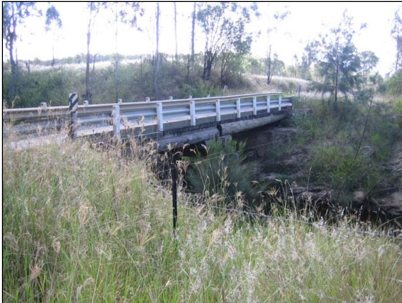
Photo 3 Ripley Road Bridge
