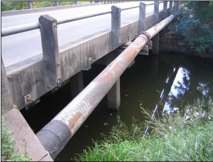
Photo 2 Swanbank Road Bridge
