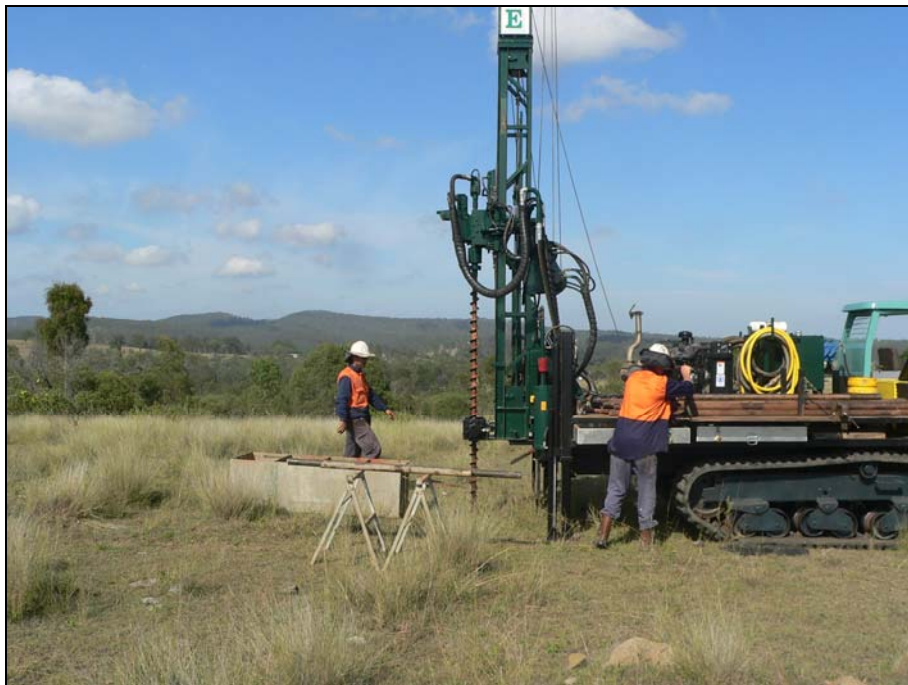
PLATE 1: TYPICAL SITE VIEW SHOWING DRILL RIG IN OPERATION
