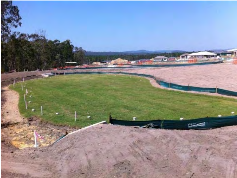
Photo: Bioretention B1a (Precinct 1) with protective turf during building phase
