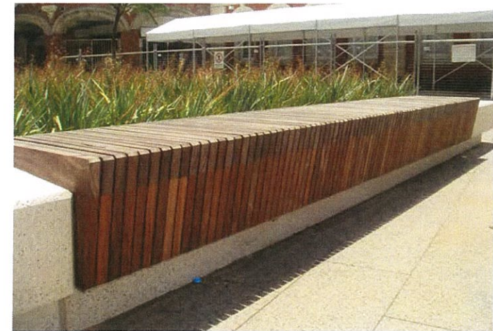
Timber seat detail to top of wall
