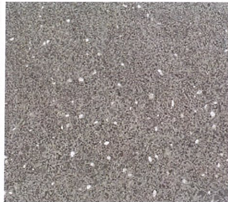
P6: Car park footpath treatment
