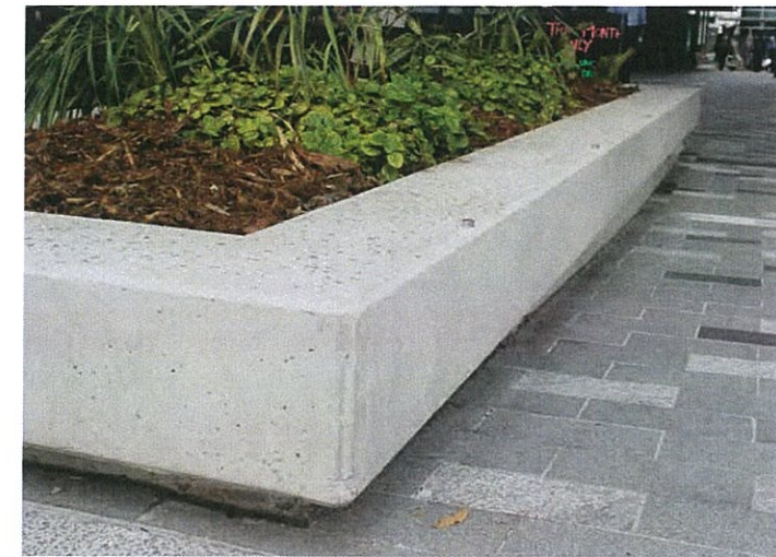
Off form uncoloured concrete landscape wall with feature aggregate and honed top finish
