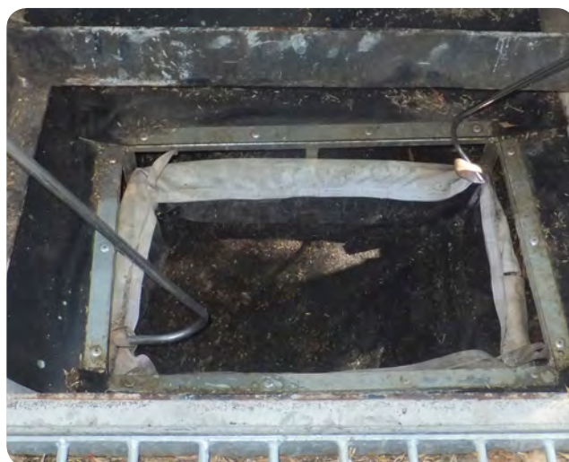
Photo 21 Correctly installed filter bag
