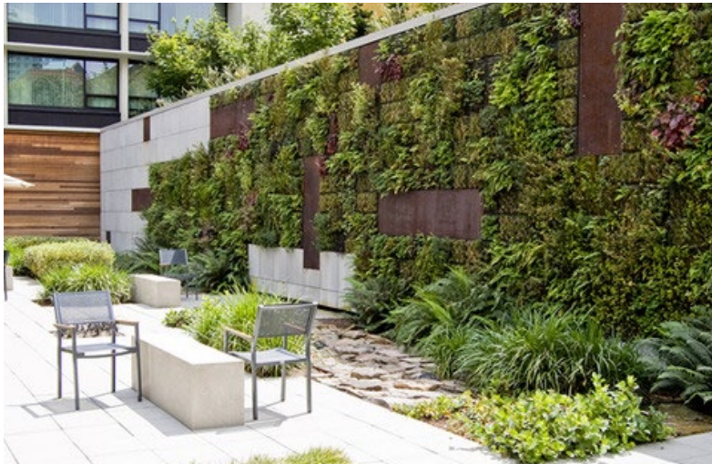
Detailed soft + hard finishes to walls
