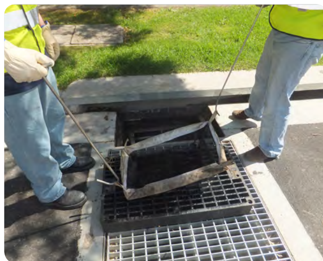
Photo 19 Reinstall filter bag
