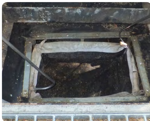
Photo 21 Correctly installed filter bag
