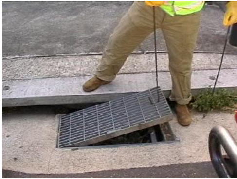
Plate 2 Lifting the grate
