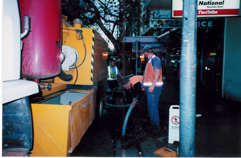
Plate 11 Cleaning an Enviropod using the inductor method
