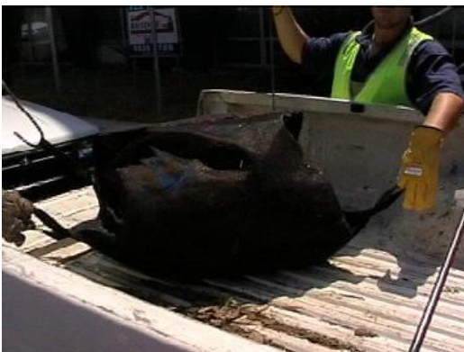
Plate 16 Grab the bottom lifting loops
