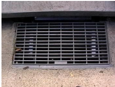
Plate 23 Installed filter bag and sealed pit
