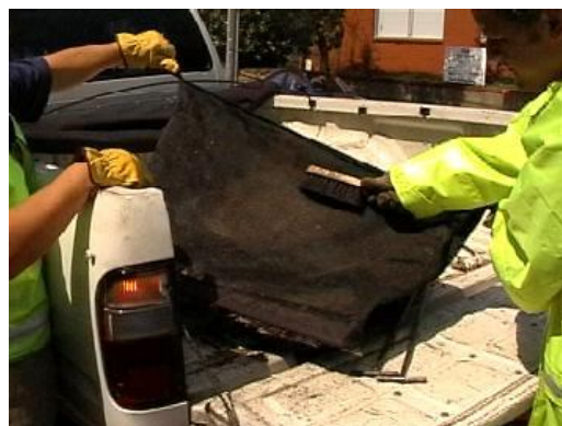
Plate 19 Brush the pores filter bag with a
