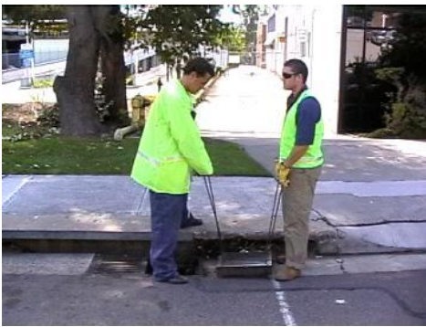
Plate 8 Lift grate and move grate to one side
