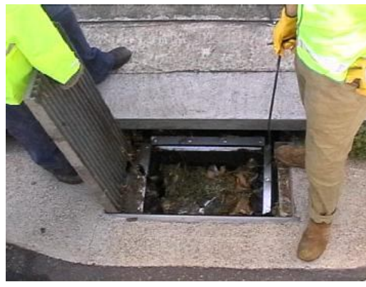
Plate 13 Lift the bag from the cage and support frame
