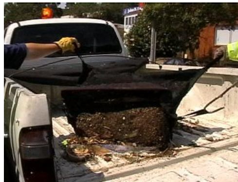
Plate 17 Lifting the bottom bag loops empty the filter bag
