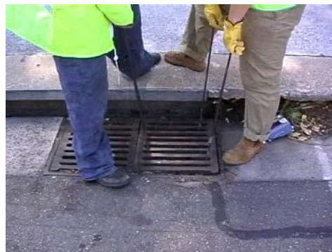
Plate 7 Position each lifter either side of the grate
