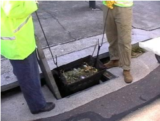
Plate 14 Lift the bag from the stormwater pit
