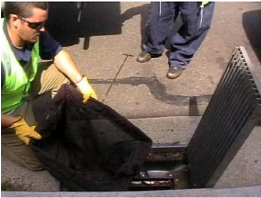
Plate 20 Reinstall filter bag
