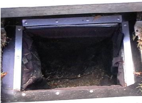
Plate 22 Correctly installed filter bag
