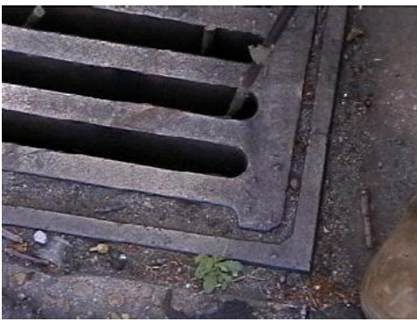
Plate 6 Insert hook near edge of grate
