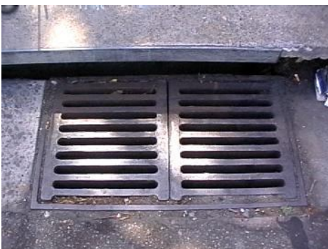
Plate 10 Reinstated non hinged grate
