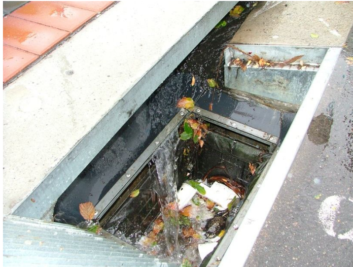
Enviropod filter in service.
