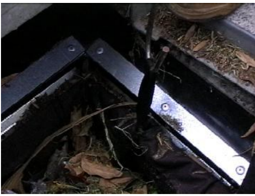
Plate 12 Place the lifting hooks through the bag loops
