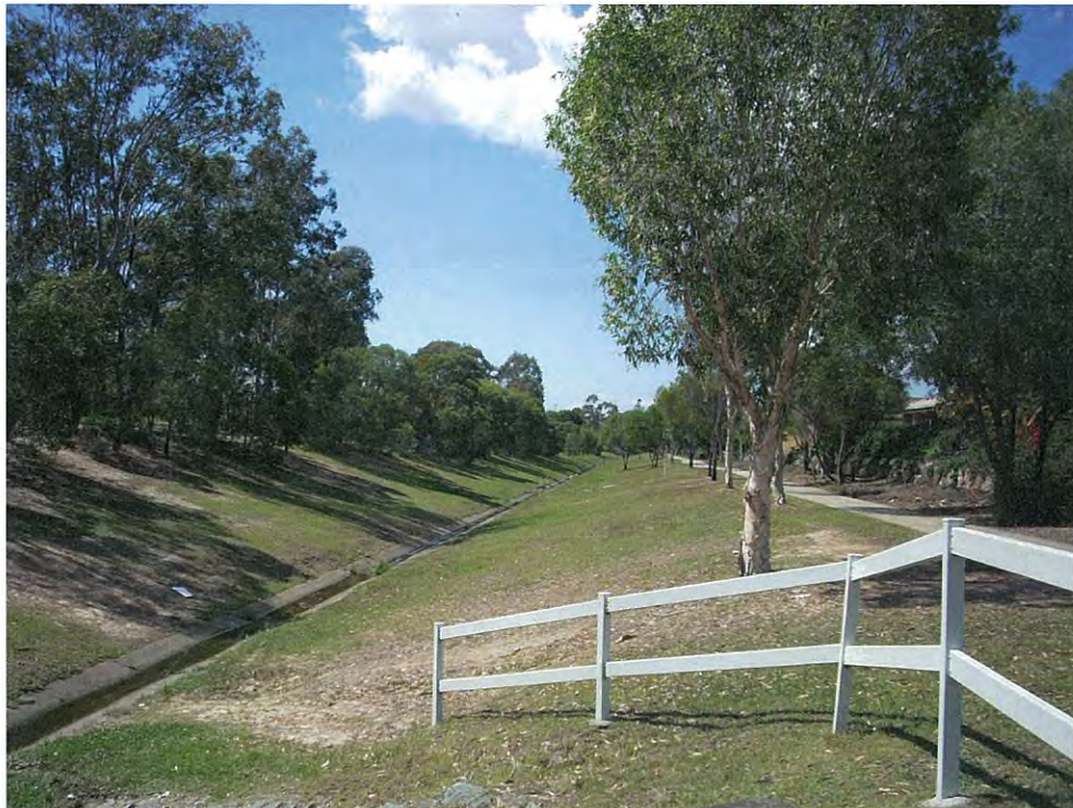
Figure 2.4 Photograph of Fitzgibbon Drain
