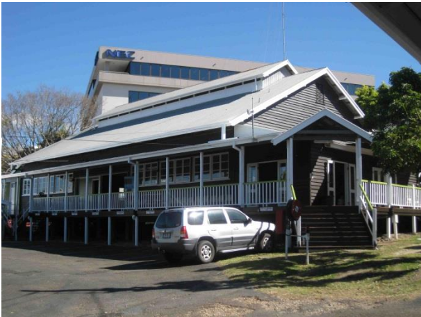
PICTURE 1 – THE FORMER DRILL HALL – SOUTHERN ELEVATION
