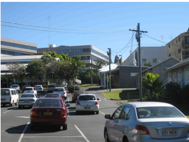
PICTURE 3 – THE WIDER VIEW OF THE FORMER ARMY DEPOT SITE, WITH THE BUILDINGS ON THE SUBJECT SITE IN THE BACKGROUND
