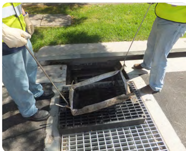
Photo 19 Reinstall filter bag
