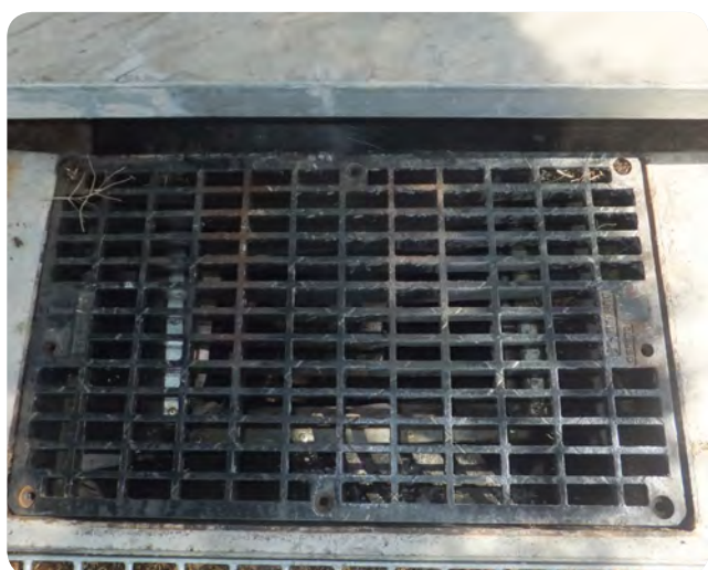
Photo 22 Installed filter bag and sealed pit
