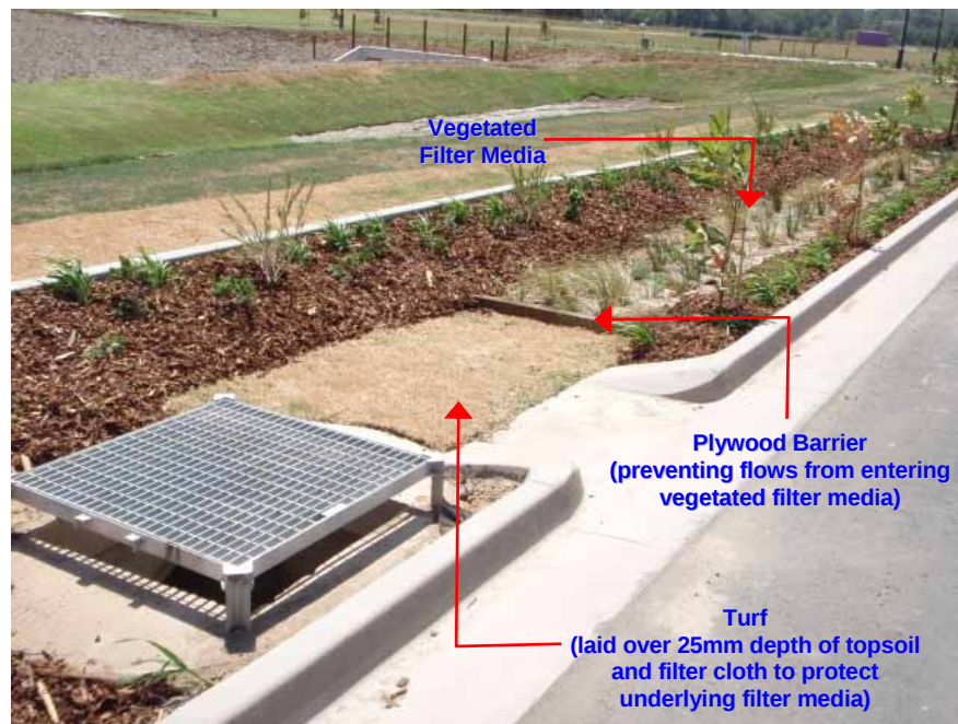
Figure 2-6 Example of Streetscape Bioretention System with Temporary Protection (During Lot-Scale Works)
