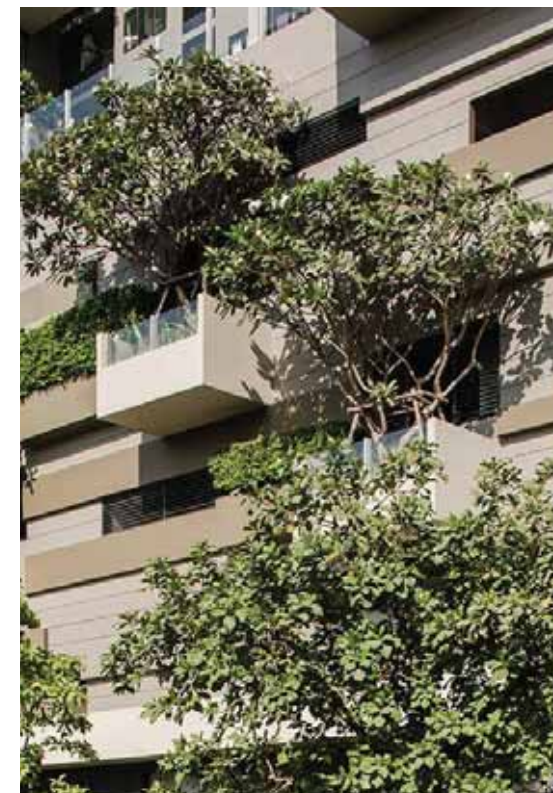
modular gardens to fill the vertical face of the built form and act as respite spaces
