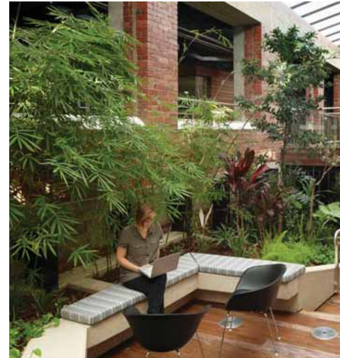
FORMED CONCRETE AND NATURAL TIMBER SEATING ELEMENTS FOR BOTH SCULPTURE AND FUNCTION
