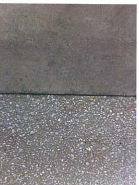
Exposed Agg concrete
