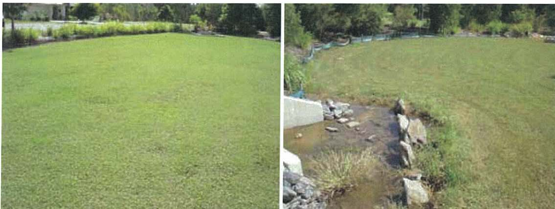
Figure 3-5 Example of a Bioretention Basin with Temporary Protection (During Lot-Scale Works)
