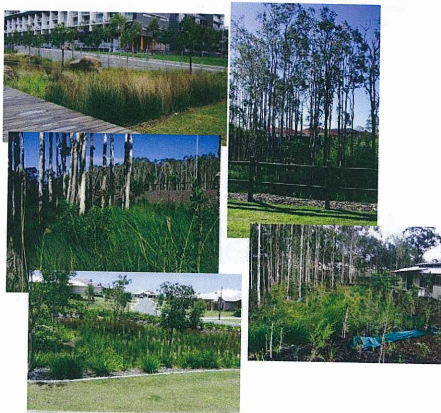
Figure 14 Examples of bio-retention in urban settings
