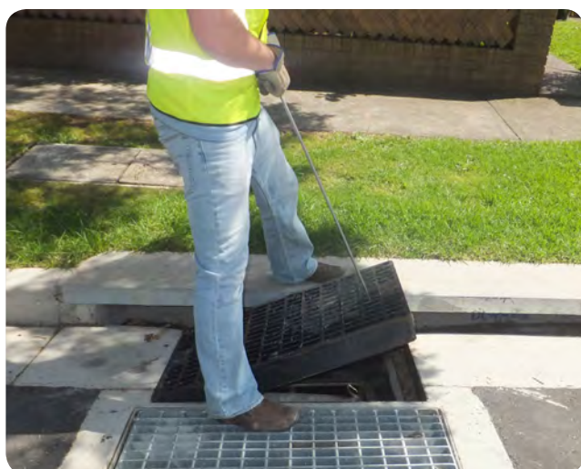
Photo 3 Lifting the grate
