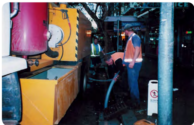
Photo 11 Cleaning an EnviroPod using the inductor method
