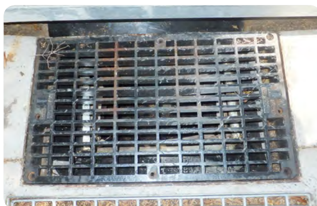
Photo 10 Reinstated non hinged grate
