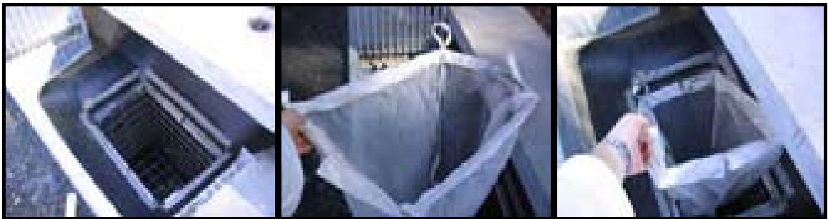
Figure 3-7 Pictures of Gully Baskets and Filter Mesh Installation
