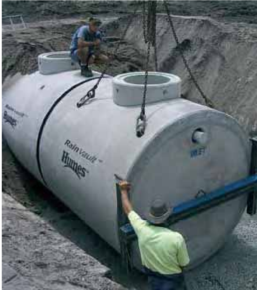
Figure 3-10 Installation of an Underground Stormwater Harvesting Tank
