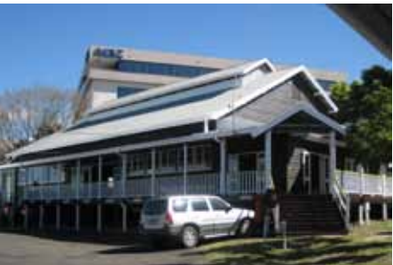
10. The Drill Hall
