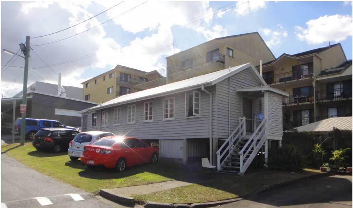
Photo 9: The ca. 1940s/1950s model ward building.
