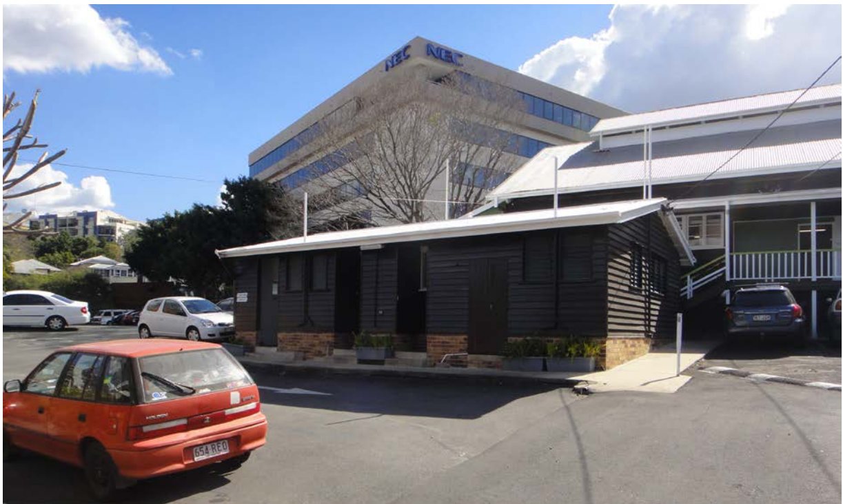
Photo 8: The 1950s toilet.
