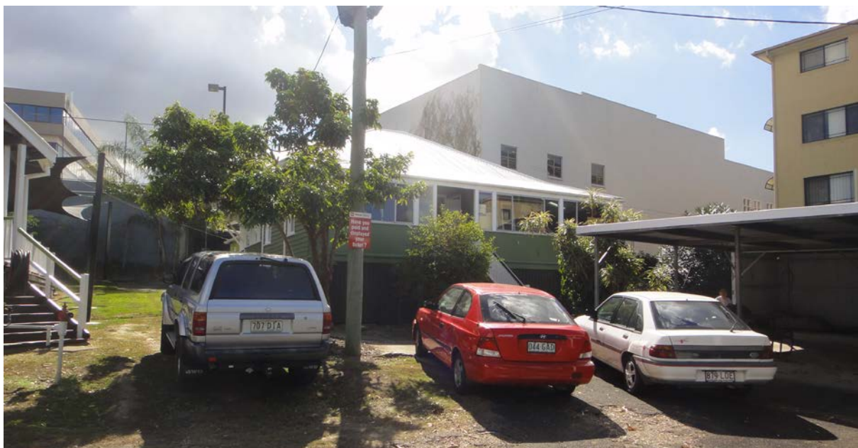
Photo 3: The nineteenth century former caretaker's cottage.
