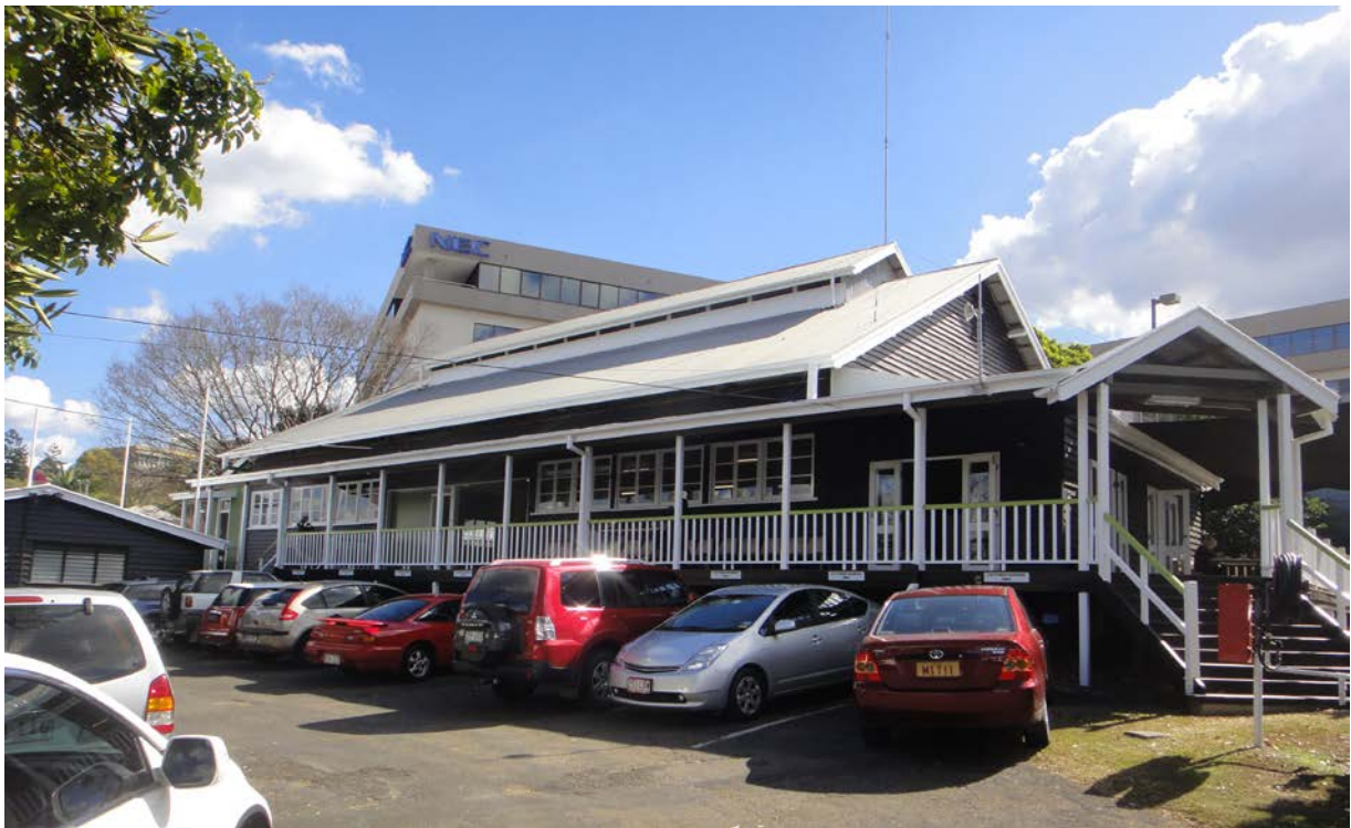
Photo 2: The 1884 former drill hall.
