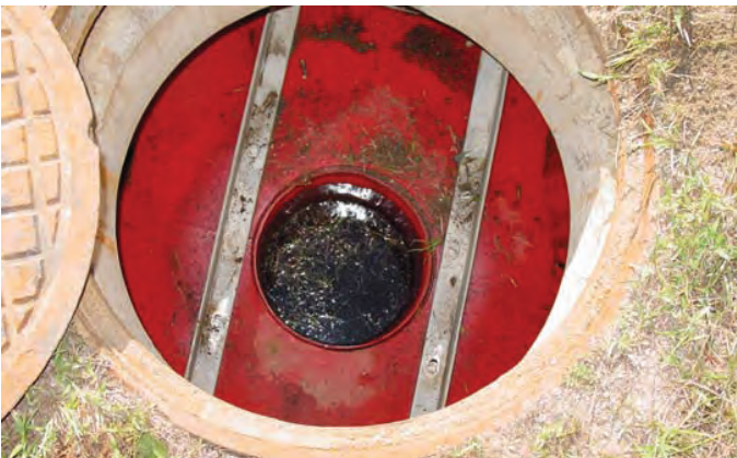
Figure 6: View over Center Shaft into sediment storage Zone
