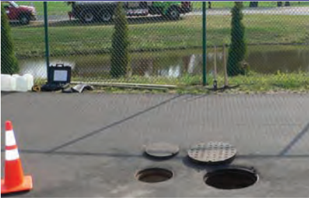
Figure 3 – Inspection and Maintenance Covers
