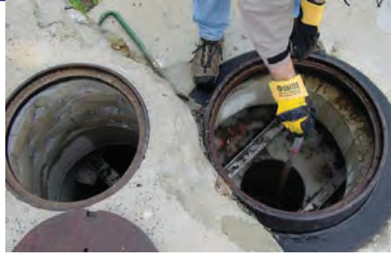
Figure 4 – Checking Sediment using a Probe
