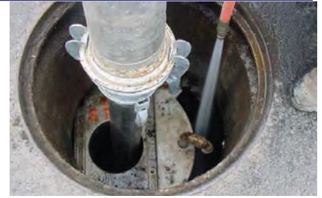
Figure 5 – Vacuuming Sediment Sump
