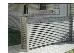
REFUSE BIN ENCLOSURE ALUMINIUM SCREENS H = 1.80m
