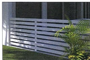
TYPE 2 Timber Fence, H = 120 cm 25% Transparency
