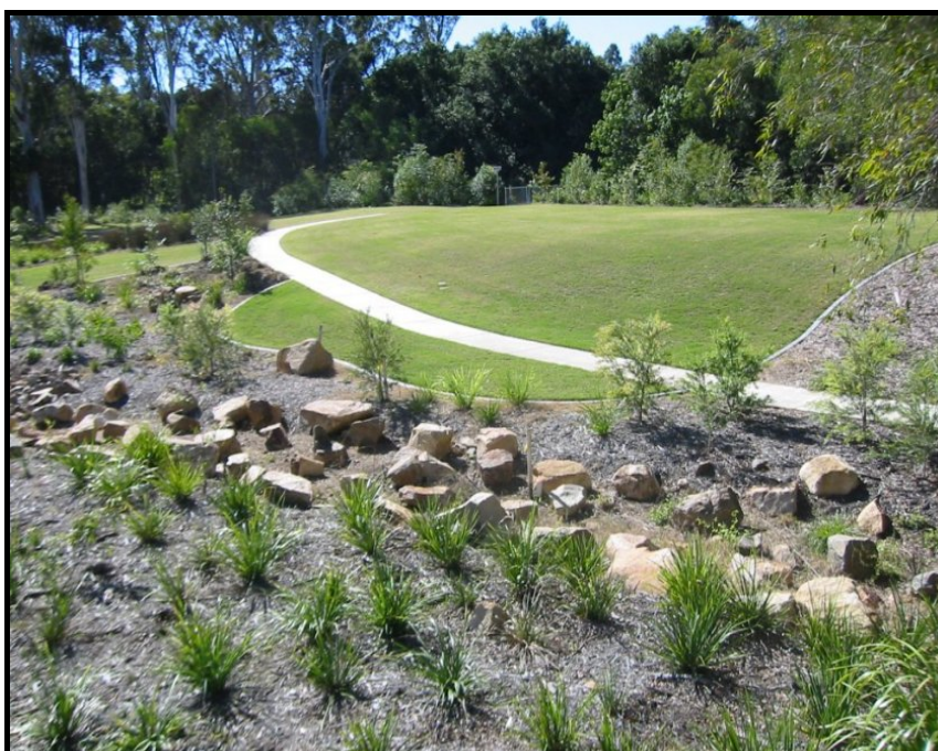
Figure 2- Typical Bioretention Basin
