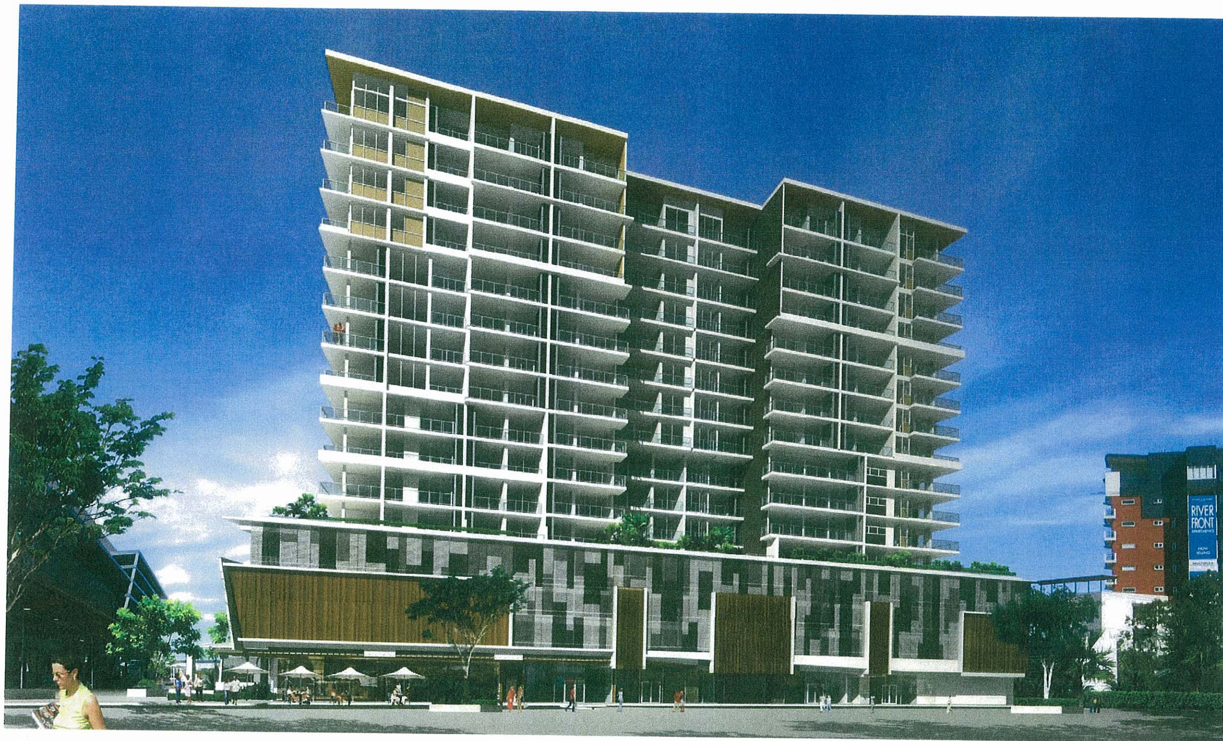
VIEW FROM NORTH
