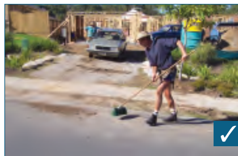
Undertake regular site clean-ups
