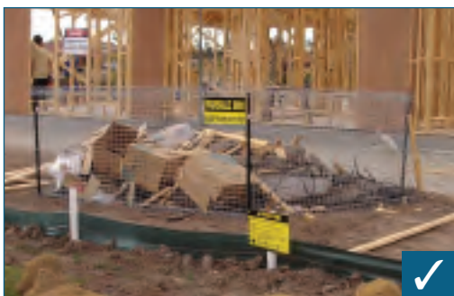
One way to properly store building waste
