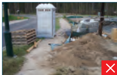
Poor site planning – stockpile over sediment fence, materials and toilet stored outside building site
