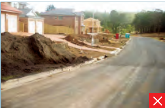
Stockpiles without protection
