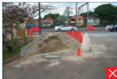
Don't store stockpiles on hard surfaces without suitable protection
