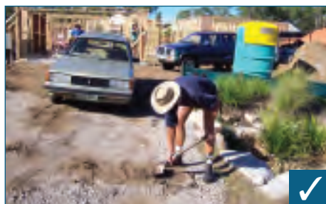
Excessive sediment deposits must be removed from entry/exit point (rumble pad) and additional crushed rock applied
