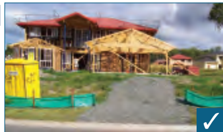
Stabilised gravel entry/exit point (rumble pad)
