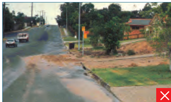
Mud and dirt on road after rain due to poor on-site erosion and sediment control
