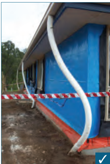
Temporary roof water connection
