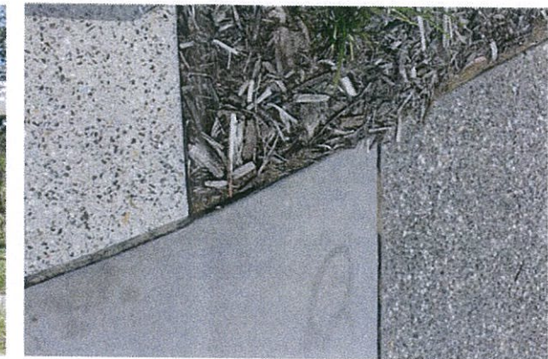
Typical exposed aggregate and oxide coloured concrete to be used in feature paving areas, eg beneath picnic shelters and furniture.
