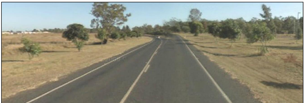
Figure 3-2: Goonyella Road looking north-west towards Moranbah (Google Street View, April 2008)
