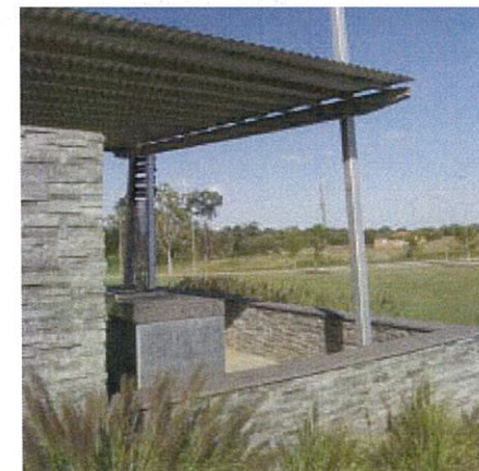
GALVANISED STEEL AND TIMBER STRUCTURE
