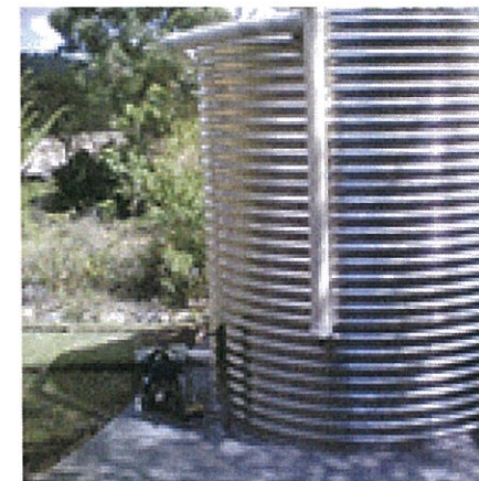
STAINLESS WATER TANK
