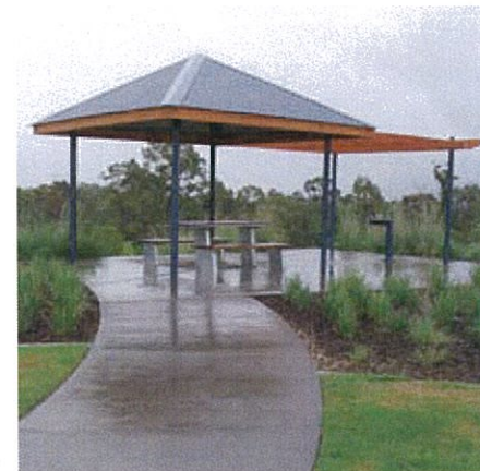
GALVANISED STEEL AND TIMBER STRUCTURE
