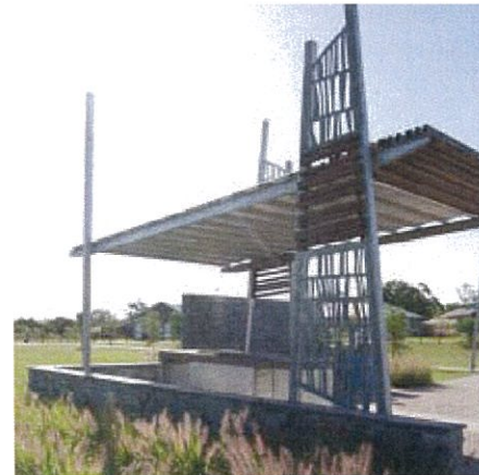
GALVANISED STEEL AND TIMBER STRUCTURE
