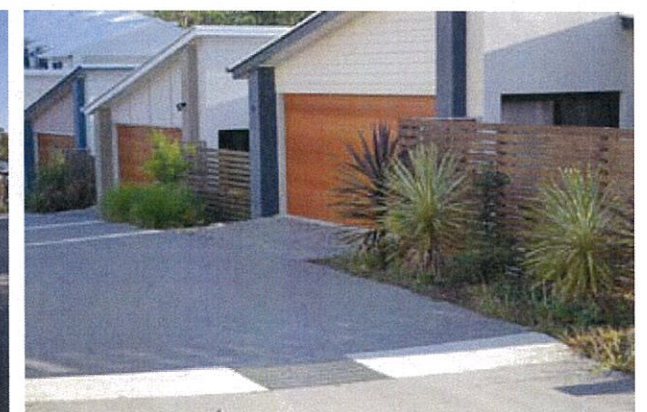
Photo illustrating planted and fenced treatment to laneway property boundary.
