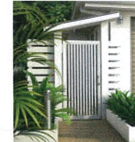
FEATURE GATE HOUSE
