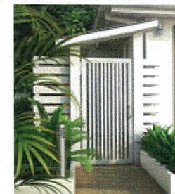
FEATURE GATE HOUSE
