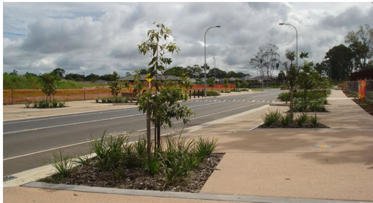
EXISTING STREET CHARACTER
