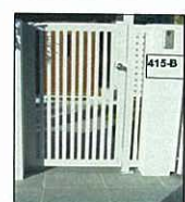
ALUMINIUM FEATURE GATE HOUSE NUMBERED 415B
