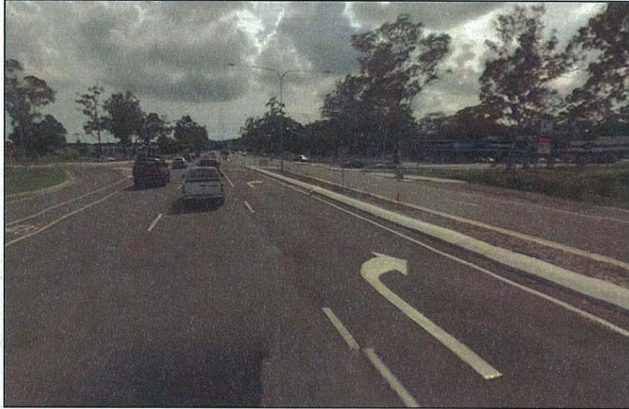
Figure 2.5 Dawson Highway (East of Harvey Road Roundabout)
