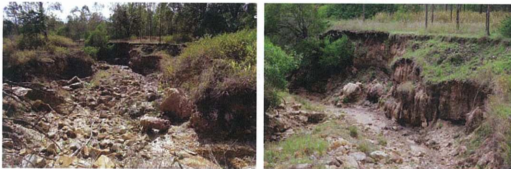
Figure 5: Active channel erosion upstream of Precinct A
