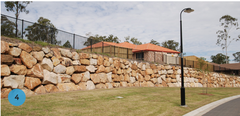
Existing retaining walls along entry experience require additional planting to increase the sense of arrival through a ‘natural setting’. Tree planting will provide a visual barrier into the rear of the residential allotments from the street.
