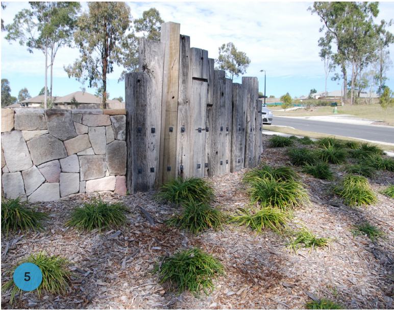
Existing entry into the site using sandstone and timber will remain as it supports the broader landscape character of the site.
