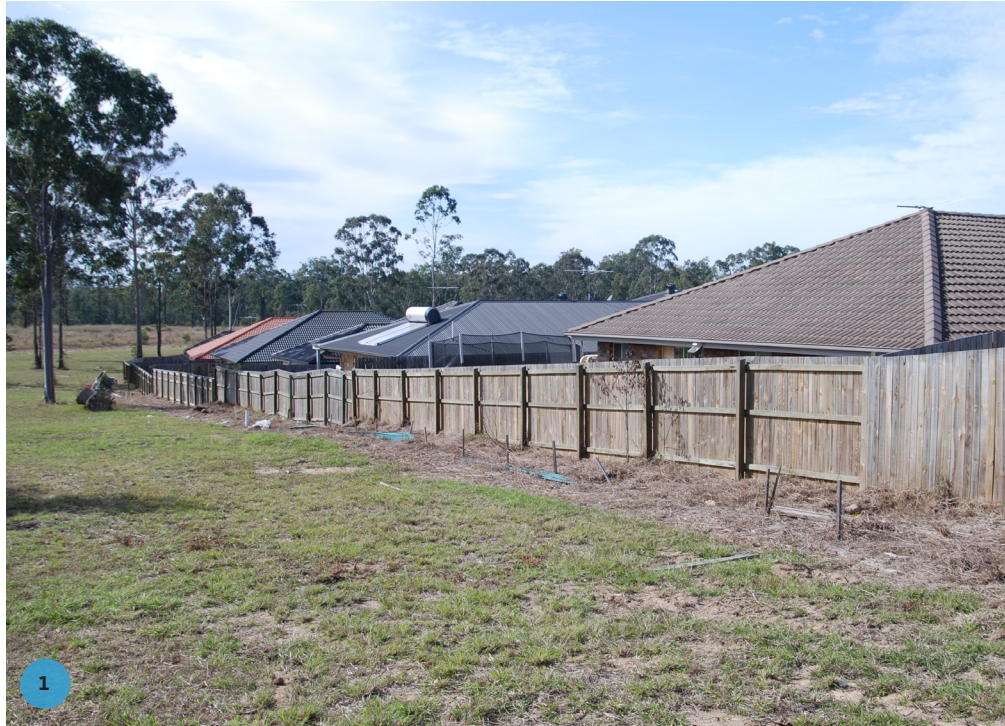
Rear fence interface with existing houses
