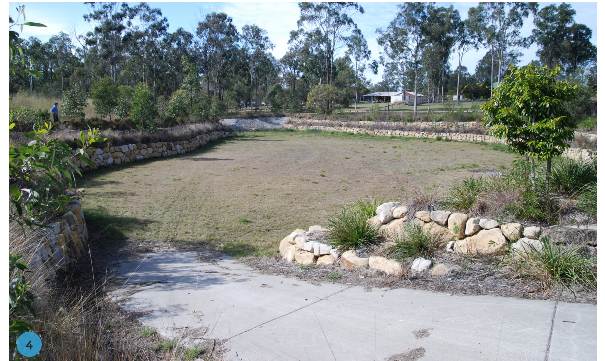
The stormwater retention basin on the southern edge of the site
