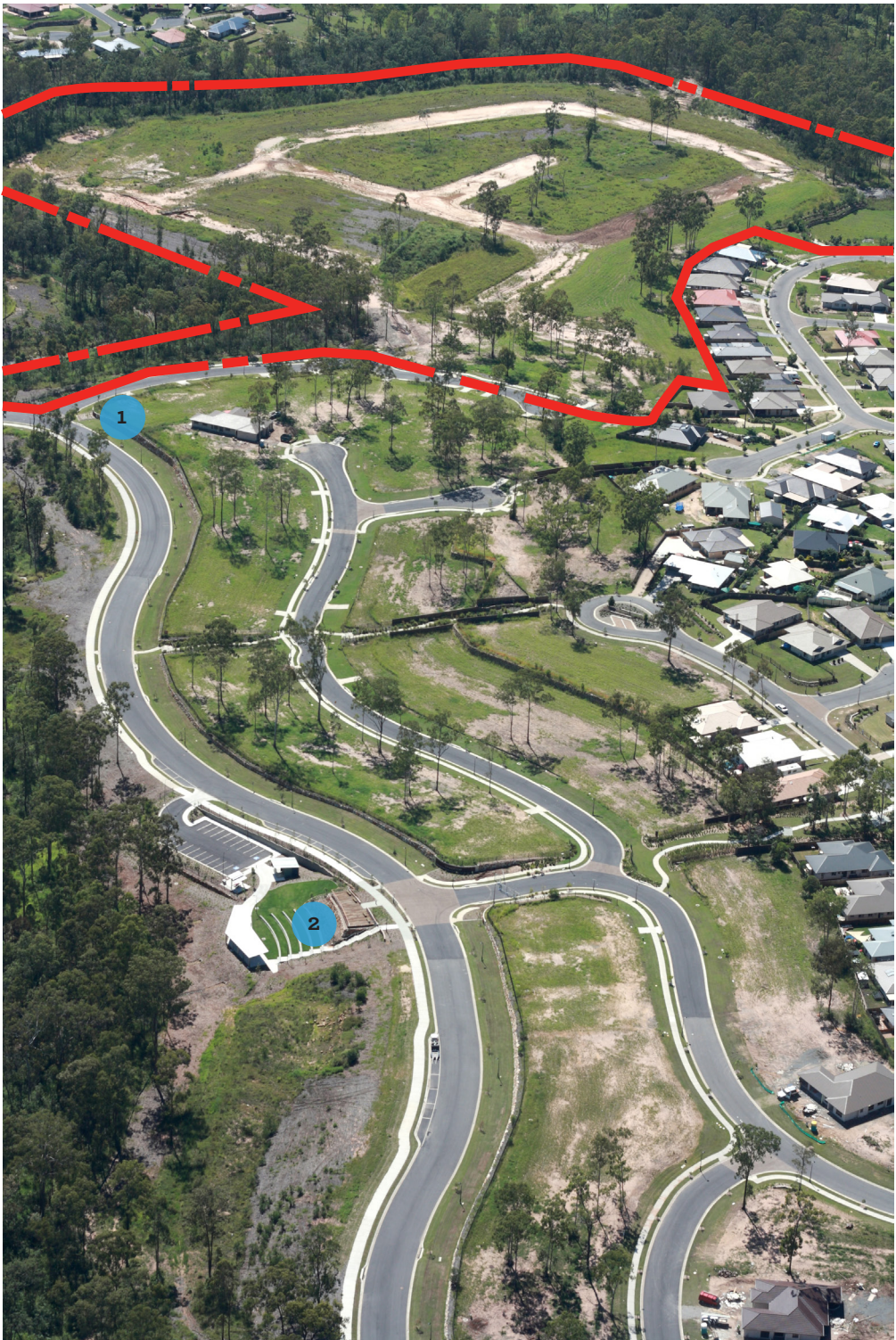
An aerial of Parkside Drive showing the district open space (left), new housing (right) and the site (top)
