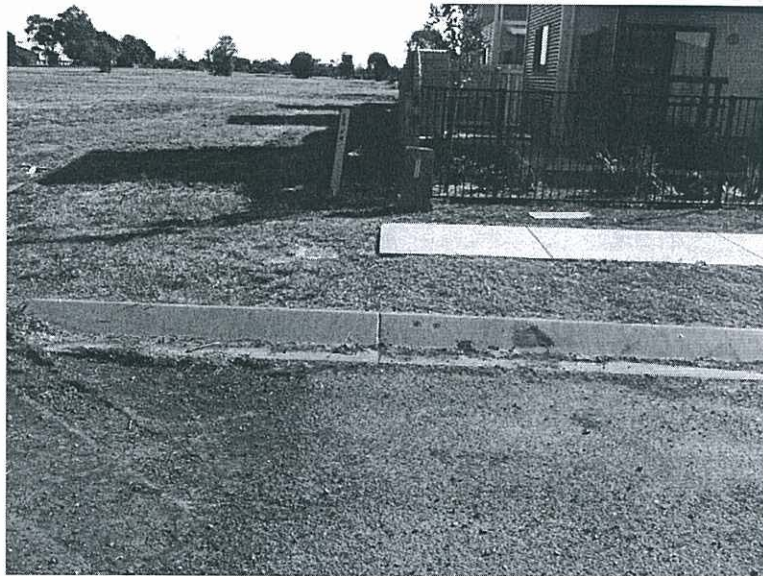
Figure 8 – Nearest telecommunication installation at Deacon Drive
