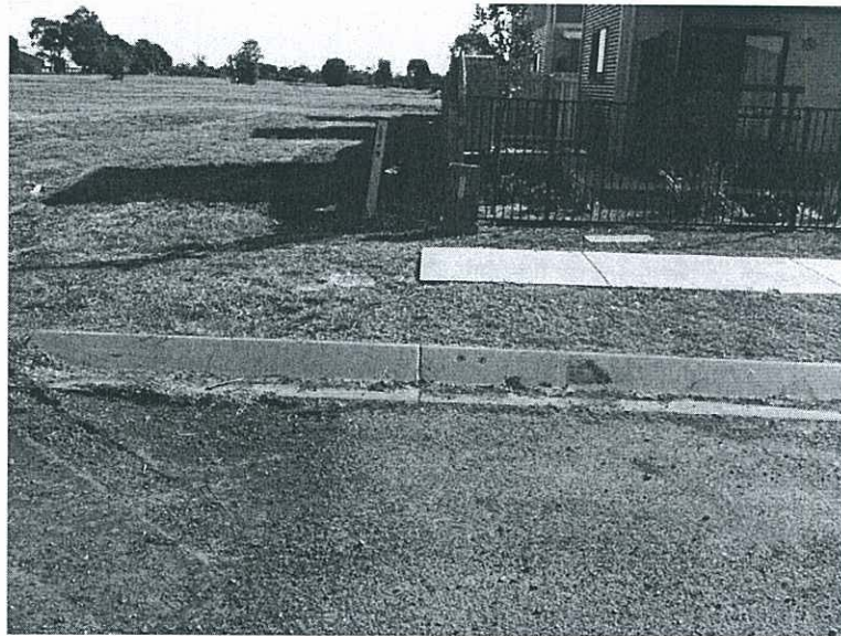
Figure 5 – Fire Hydrant at end of Deacon Drive
